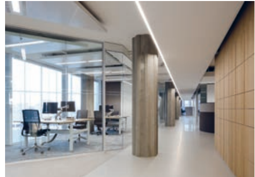
The building's interior has been completely transformed, but its concrete structure, complete with its characteristic octagonal columns, is still there and visible.
