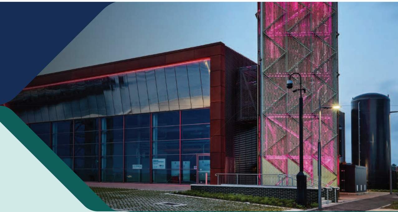
Queens Quay Heat Network. Picture: West Dunbartonshire Council
