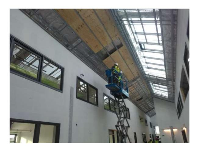
Photograph of ceiling install showing underside of cassette, MF ceiling rails and plywood pattressing.
