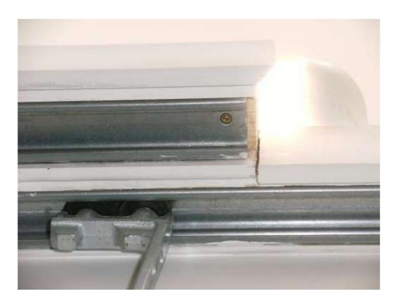
Photograph showing the overlapping top rails and missing stopper.
